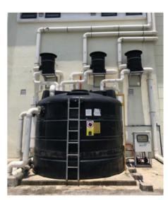
➤ A rain harvesting system with storage capacity of 13,500 litres is used for site washing and plant watering at Langat CSTP
